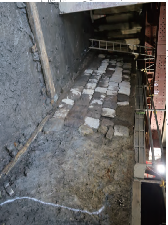
①北横仕切堤石垣撤去状況-1 (2022. 10.24)
