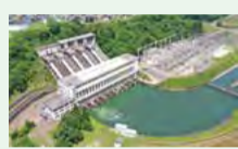
信濃川水力発電所 Shinanogawa Hydroelectric Power Plant
