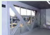
【駅舎補強】 [Seismic reinforcement to station building]
