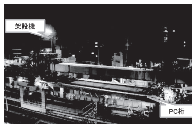
(c) PC桁架設状況
