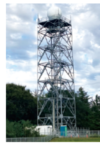
Doppler radar installed at Kuromori, Sakata
