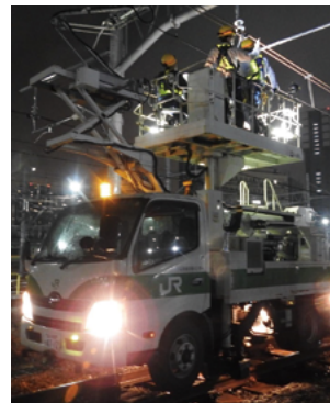
Overhead wire inspection work
