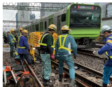
Construction work during daytime hours (Keihin-Tohoku Line)
