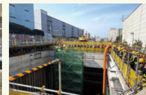
IR Day (Haneda Airport Access Line (tentative name) Project Site Visit)
