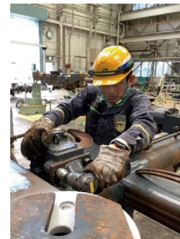
Unit brake installation work on truck frames by technical interns
