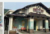
A store using the station building (Atami Purin Kinomiya Station Store)
