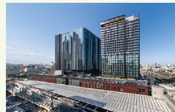
Full view of OIMACHI TRACKS
