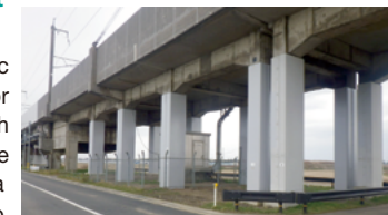
Seismic reinforcement of elevated railway tracks
