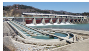
Construction of fishways (Miyanaka Intake Dam)
