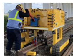
Mechanization of rail replacement work
