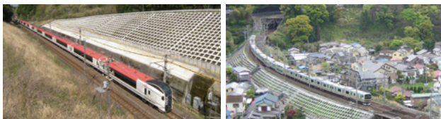
Cutting slope protection (spray framework)
