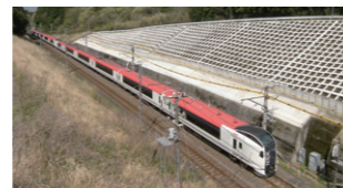
Cutting slope protection (spray framework)
