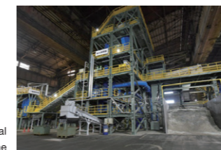
Chemical recycling raw material production line
