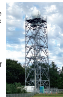
Doppler radar installed at Kuromori, Sakata
