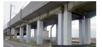
Seismic reinforcement of elevated railway tracks
