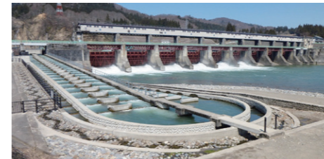
Construction of fishways (Miyanaka Intake Dam)
