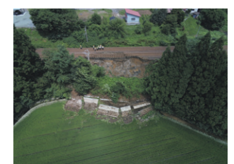
Ascertaining damage using drones
