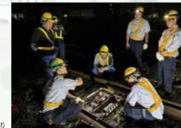
Technical support for railway maintenance (Photograph left and right)
