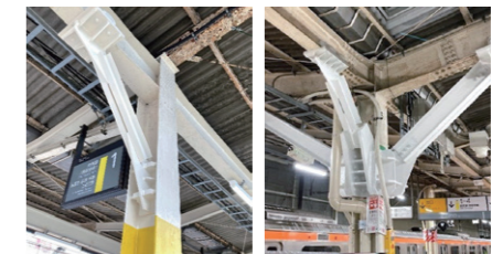
Smart Weak Axis Method (Photograph on left) Smart Both Axis Method (Photograph on right)
