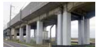
Seismic reinforcement of elevated railway tracks
