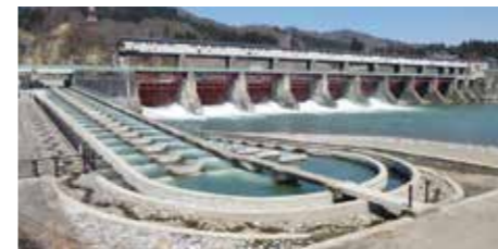
Construction of fishways (Miyanaoka Intake Dam)
