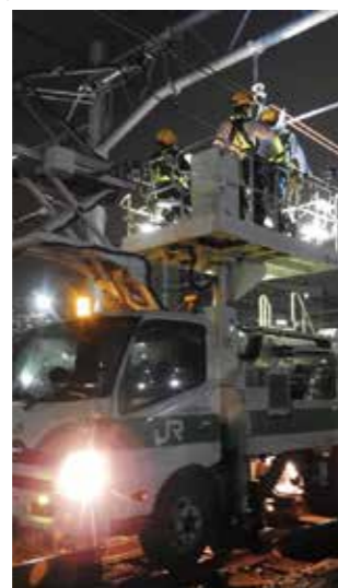
Overhead wire inspection work
