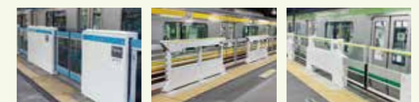
Conventional platform gates Slit-frame platform doors Smart Platform Doors®
