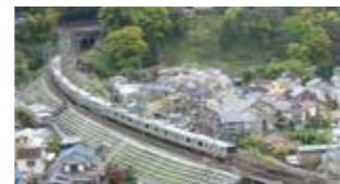
Embankment slope protection (spray framework)
