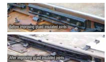
After improving glued insulated joints
