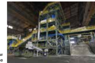
Chemical recycling raw material production line
