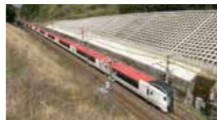
Cutting slope protection (spray framework)
