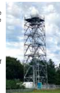
Doppler radar installed at Kuromori, Sakata
