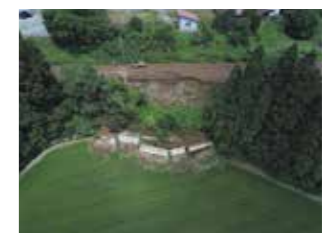
Ascertaining damage using drones
