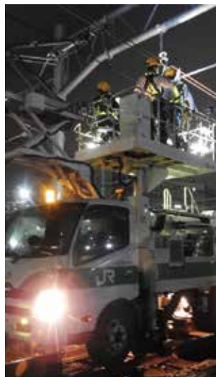
Overhead wire inspection work
