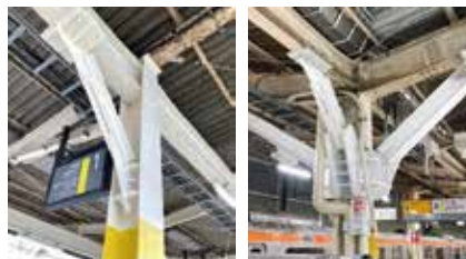
Smart Weak Axis Method (Photograph on left) Smart Both Axis Method (Photograph on right)
