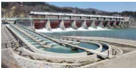
Construction of fishways (Miyanaka Intake Dam)
