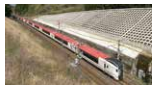
Cutting slope protection (spray framework)
