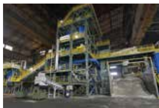
Chemical recycling raw material production line
