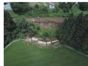
Ascertaining damage using drones
