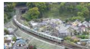
Embankment slope protection (spray framework)
