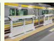
Slit-frame platform doors
