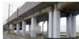
Seismic reinforcement of elevated railway tracks
