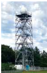
Doppler radar installed at Kuromori, Sakata
