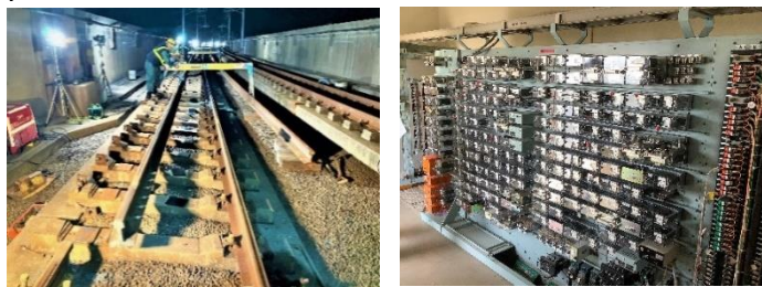
Key repair work (Left: Rail replacement; Right: Signal relay replacement)
