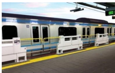
Installation of automatic platform gates
