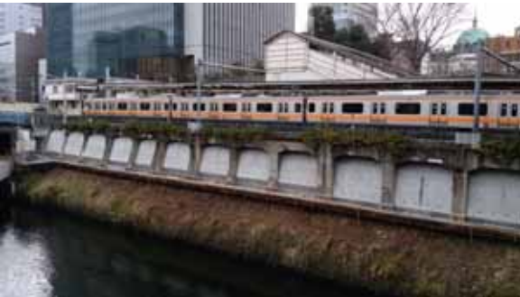
Seismic reinforcement of embankments
