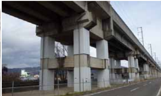
Seismic reinforcement of viaduct columns
