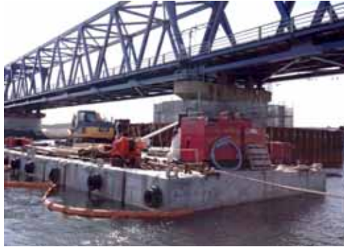
Seismic reinforcement of bridge piers
