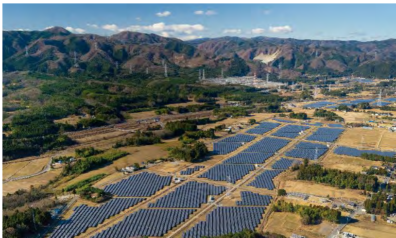
Project-04 Solar power generation
