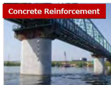
Seismic reinforcement of bridge piers
