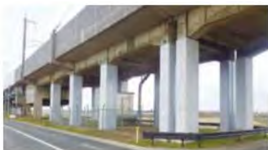
Seismic reinforcement of elevated railway tracks
