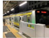
Installation of automatic platform gates
