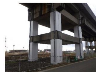
Countermeasures against large-scale earthquakes (elevated railway track pillars for Shinkansen)
