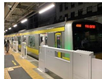
Installation of automatic platform gates
