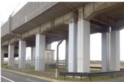
Earthquake-proofing for under railway viaduct columns
