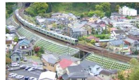
Embankment slope protection work (sprayed frame work)
