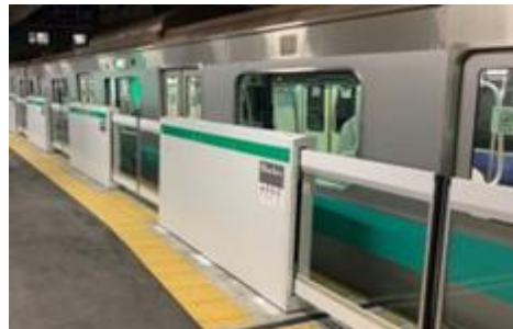
Example of platform door installation (Joban Line (local trains))
