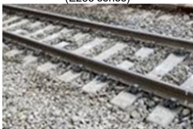
Replacing with elastic PC sleepers
