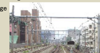
Integrated overhead contact lines
