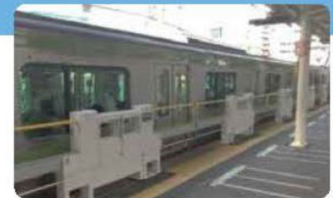
Installation of platform doors
