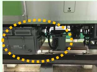
Track facilities monitoring device
