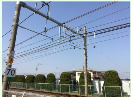
Integration of overhead wires
