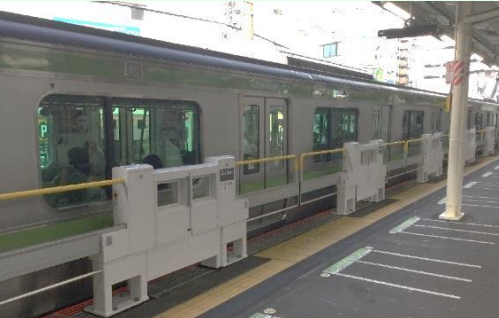
Introduction of “smart” automatic platform gates (Machida Station, Yokohama Line)
