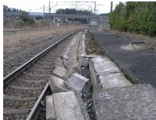
Collapse of platforms
