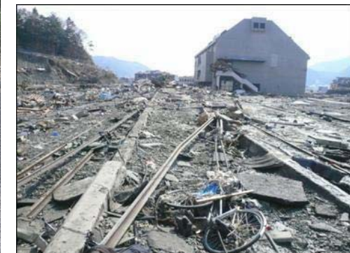
Tracks swept away
