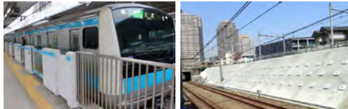
Advance of automatic platform gate installation
