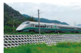
Embankment slope protection (spray-frame work)
