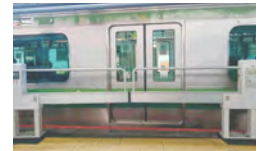
“Smart” automatic platform gates at Machida Station
