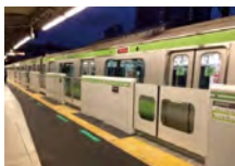
Installing automatic platform gates
