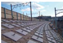
Implementing seismic reinforcement
