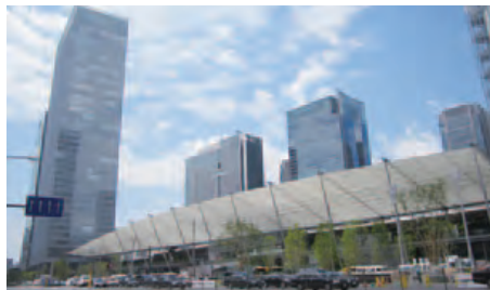
GranRoof and station-front plaza to the Yaesu entrances
