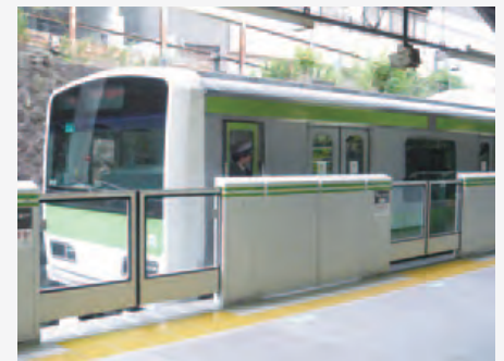
ID Automatic platform gates on the Yamanote Line
