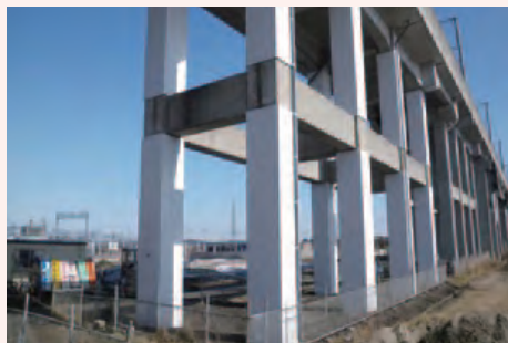
Seismic reinforcement of viaduct columns
