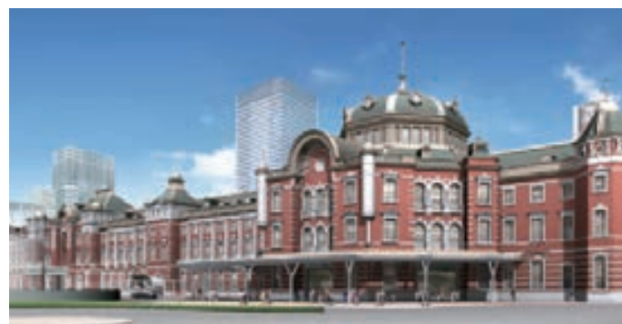
B The Tokyo Station Hotel
