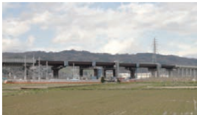
B Work to extend the Hokuriku Shinkansen Line
