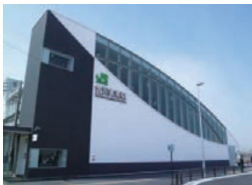
A Yoshikawaminami Station
