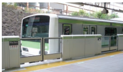
Automatic Platform Gates
