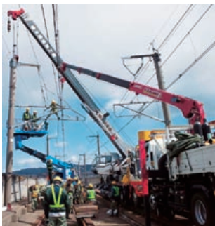
Restoration work for collapsed electric poles on the Tohoku Shinkansen Line
