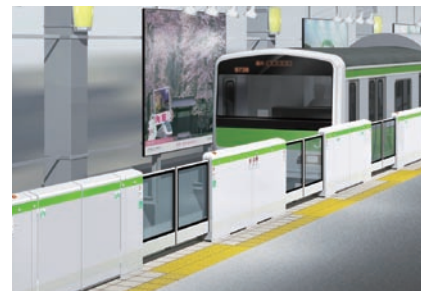
Automatic platform gates (image)
