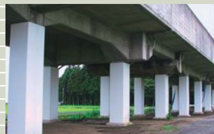
Reinforcement of supports for elevated Shinkansen tracks
