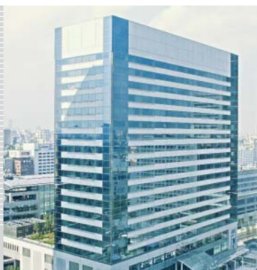
JR Shinagawa East Building
