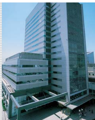
JR Tokyu Meguro Building
