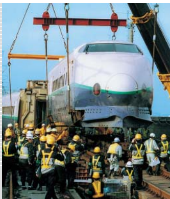
A scene of restoration work
