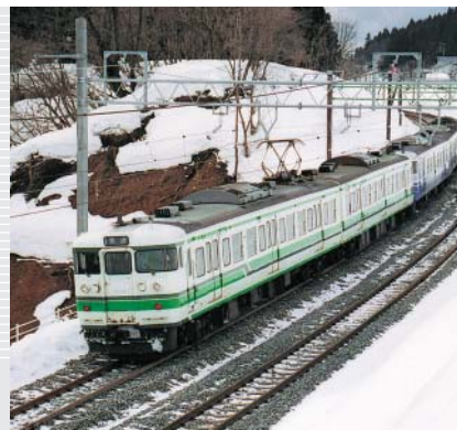
Joetsu line between Echigo Kawaguchi and Ojiya after restoration work
