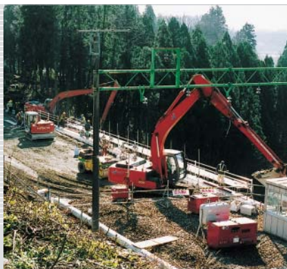
Restoration work on the Joetsu line
