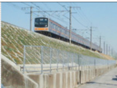
A scene of reinforced track on a conventional line
