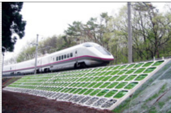
A scene of reinforced track on the Akita hybrid Shinkansen line
