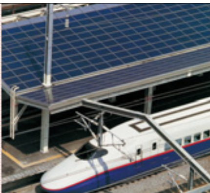
Photovoltaic generator panel at Takasaki station
