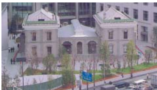
Old Shimbashi Station (Photo: Transportation News Co., Ltd.)
