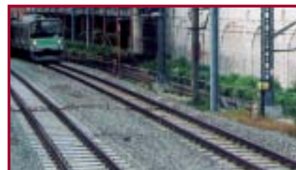
TC type low-maintenance track This track was designed to minimize labor requirements for maintenance tasks.
