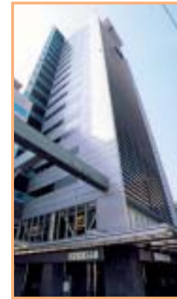
JR Tokyu Meguro Building
