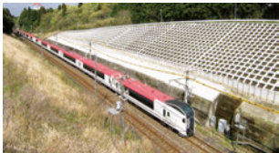
Cutting slope protection (spray framework)
