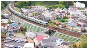
Embankment slope protection (spray framework)
