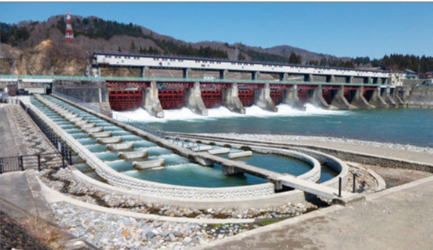
Construction of fishways (Miyanaka Intake Dam)
