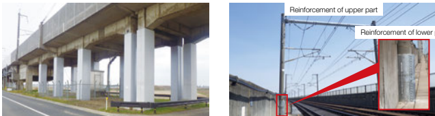
Seismic reinforcement of elevated railway tracks
