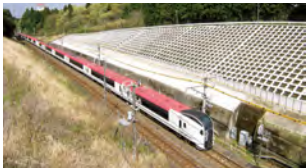
Cutting slope protection (spray framework)
