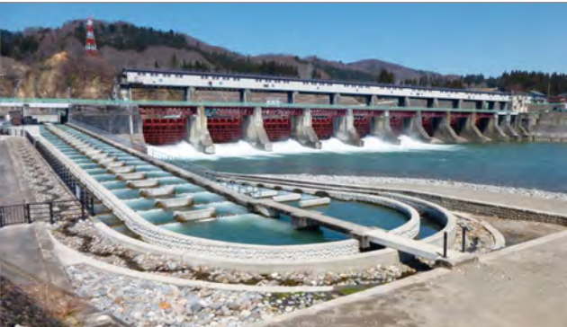
Construction of fishways (Miyanaka Intake Dam)
