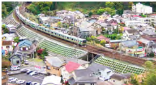
Embankment slope protection (spray framework)
