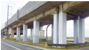
Seismic reinforcement of elevated railway tracks
