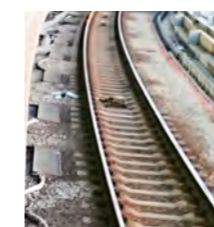
A mat placed on the tracks along the platform detects whether a person has fallen onto the tracks and notifies incoming trains to stop.
