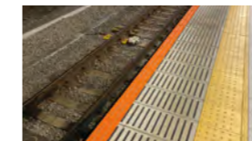
These lines use colors that people associate with danger to encourage a visual and psychological connection between danger and the platform edge.
