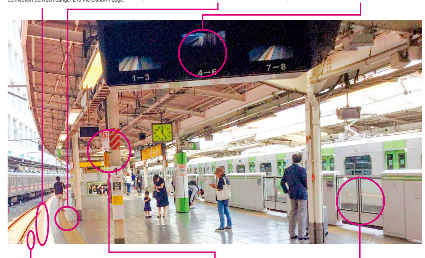
We are installing platform doors to prevent people from coming into contact with trains or falling onto tracks.
