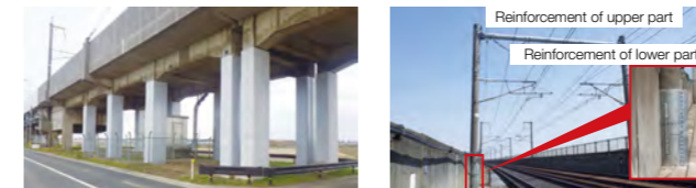
Seismic reinforcement of elevated railway tracks
