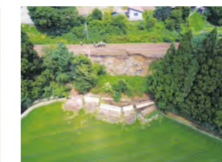
Ascertaining damage using drones
