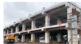
Construction of Surat Station
