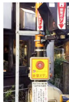
Level crossing obstacle alarm device (emergency buttons)
