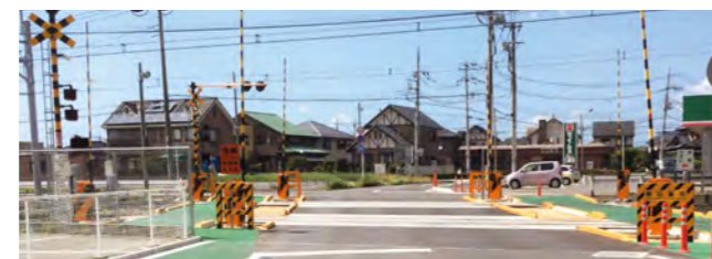
In cooperation with road administrators, we are increasing the width of level crossings and separating crossings for pedestrians from those for automobiles by making the roads and walkways different colors.
