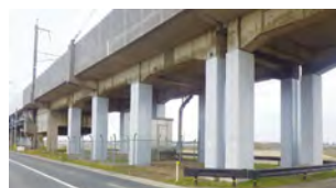
Seismic reinforcement of elevated railway tracks
