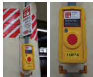
Emergency stop buttons on platforms
