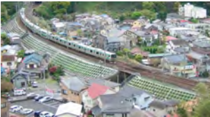
Embankment slope protection (spray framework)
