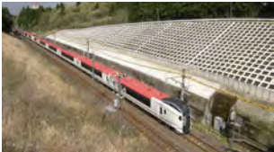
Cutting slope protection (spray framework)
