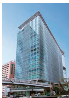
JR Minami Shinjuku Building
