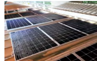
Sendagaya Station (Energy creation using solar power generation)
