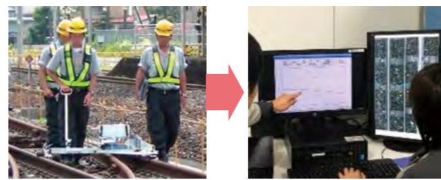
Traditional rail track inspection
