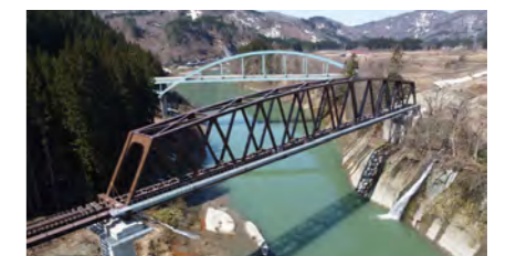
Tadami Line Restoration Work (No. 7 Tadami River Bridge)
