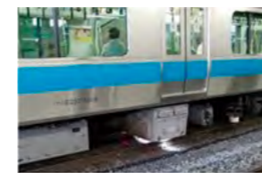
Track equipment monitoring systems (conventional lines)
