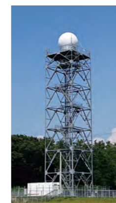
Doppler radar installed at Kuromori, Sakata
