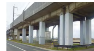
Seismic reinforcement of elevated railway tracks
