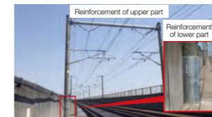
Structural reinforcement of utility poles
