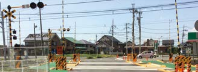
In cooperation with road administrators, we are increasing the width of level crossings and separating crossings for pedestrians from those for automobiles by changing the colors of the roads and walkways.
