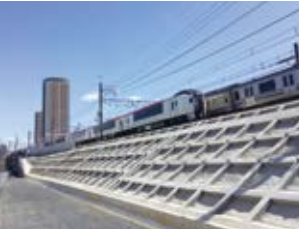
Seismic reinforcement of embankment
