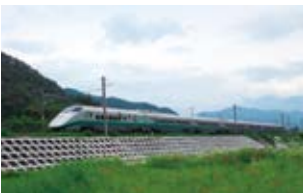
Embankment slope protection (spray framework)
