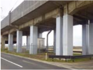
Seismic reinforcement of elevated railway tracks
