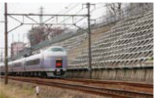
Cutting slope protection (spray framework)
