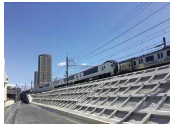
Seismic reinforcement of embankment
