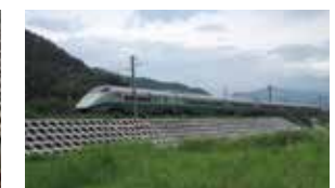
Embankment slope protection (spray frame work)
