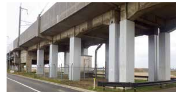
Seismic reinforcement
