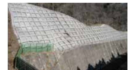
Natural slope protection (spray frame work)
