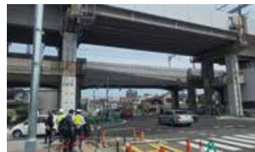
Urban planning road opened as part of continuous separated-grade crossing development
