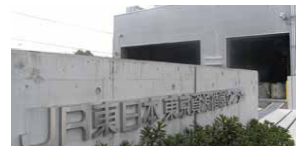
JR East Tokyo Materials Recycling Center
