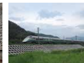
Embankment slope protection (spray frame work)
