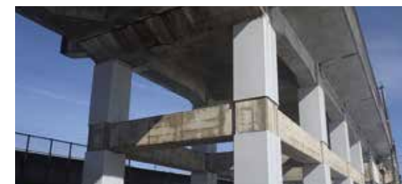
Seismic reinforcement
