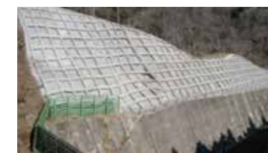
Natural slope protection (spray frame work)
