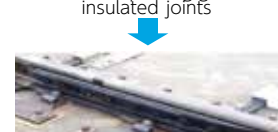
After improving glued insulated joints
