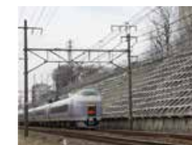
Cutting slope protection (spray frame work)
